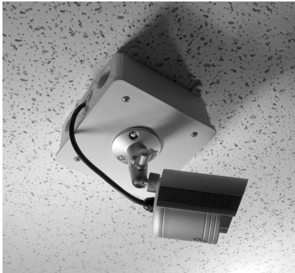
Fig. 9: Eave or Ceiling mounting
